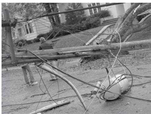
Assessing damage from Hurricane Sandy in White Plains. Thousands of homes and businesses were without power for a week or more. Photo: NY Patch
